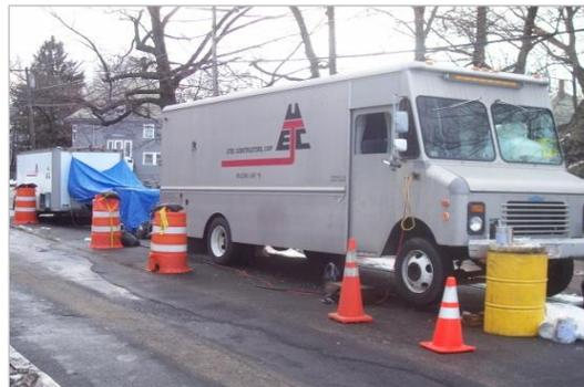
Cable splicing setup
